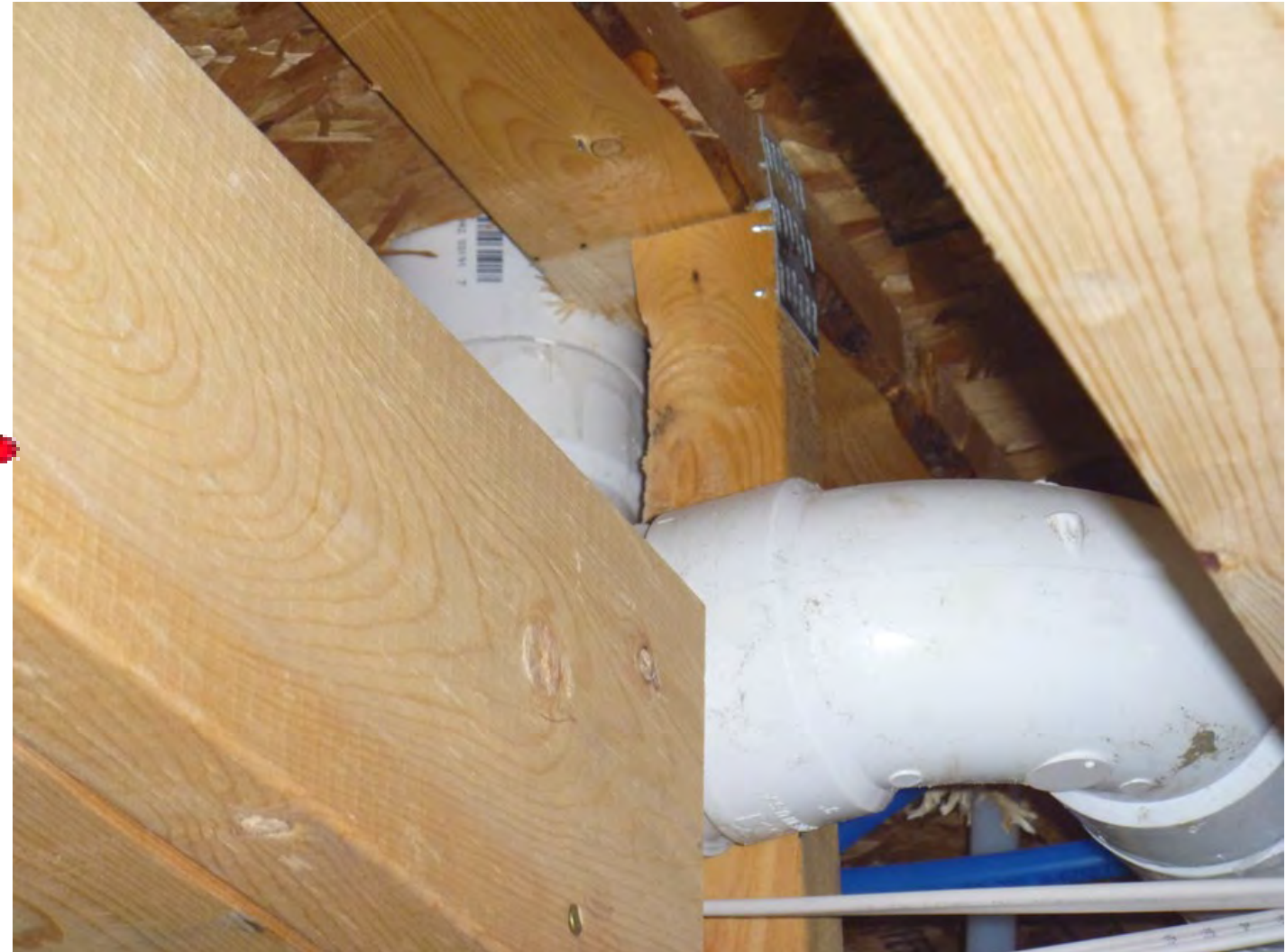
Nail plates and truss top chords are really overrated!
